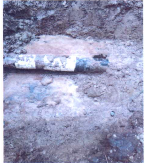
SPILL POINT AFTER EXCAVATION: fig2
