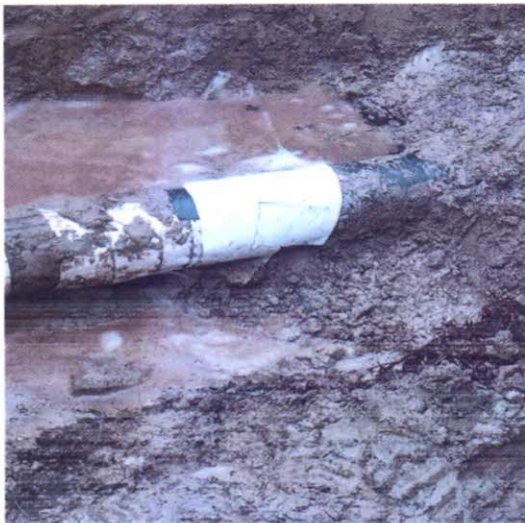
SPILL POINT AFTER REPAIRS: fig3
